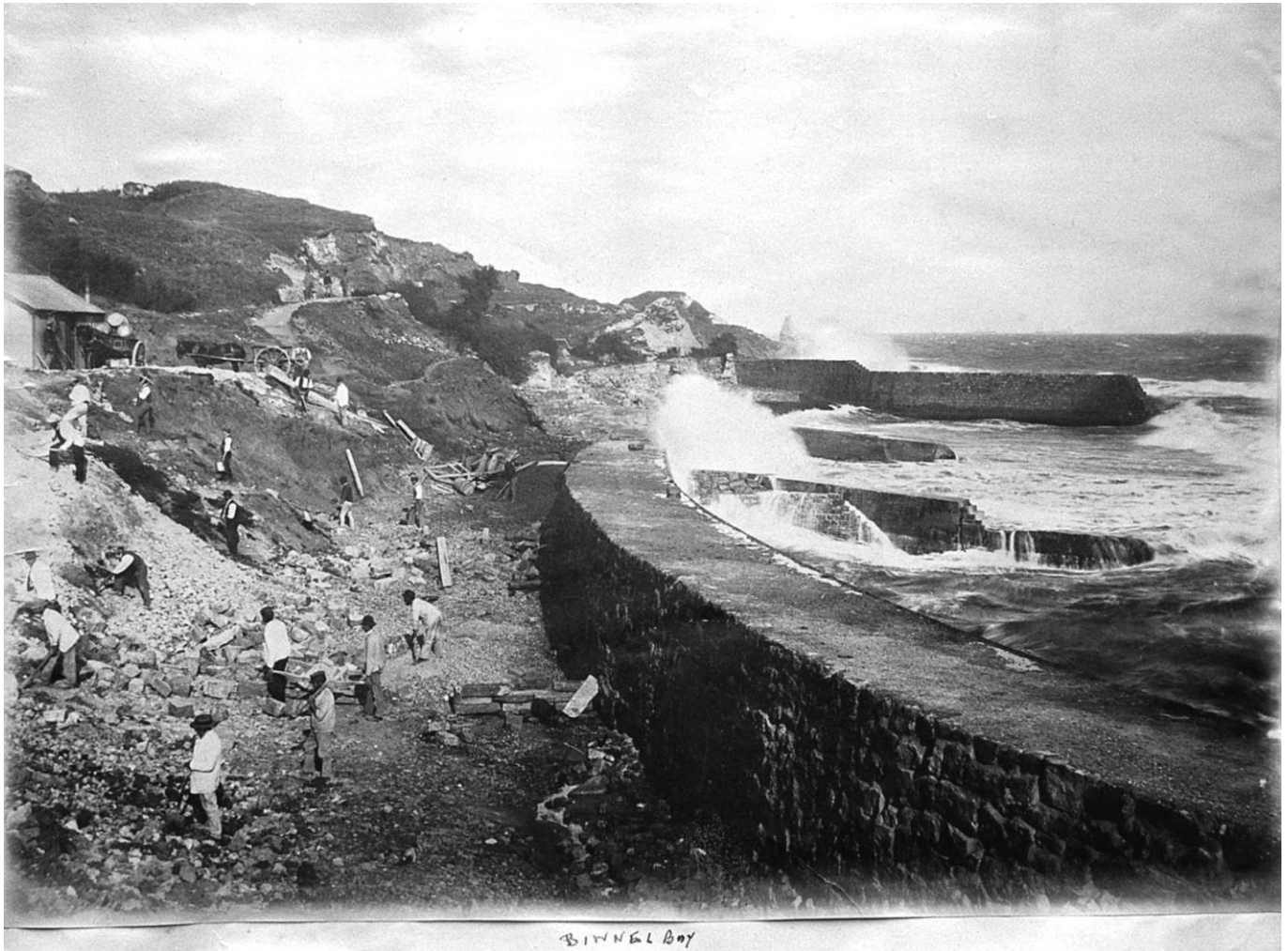
Figure IW.37.3.1 Historic harbour attempt at Binnel Bay along the Undercliff, now lost to erosion.
