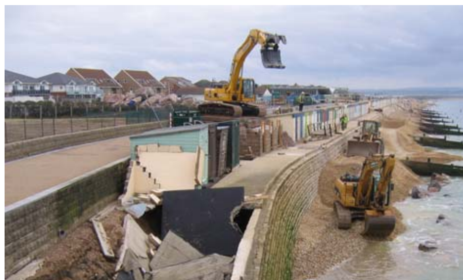
Works at Milford
