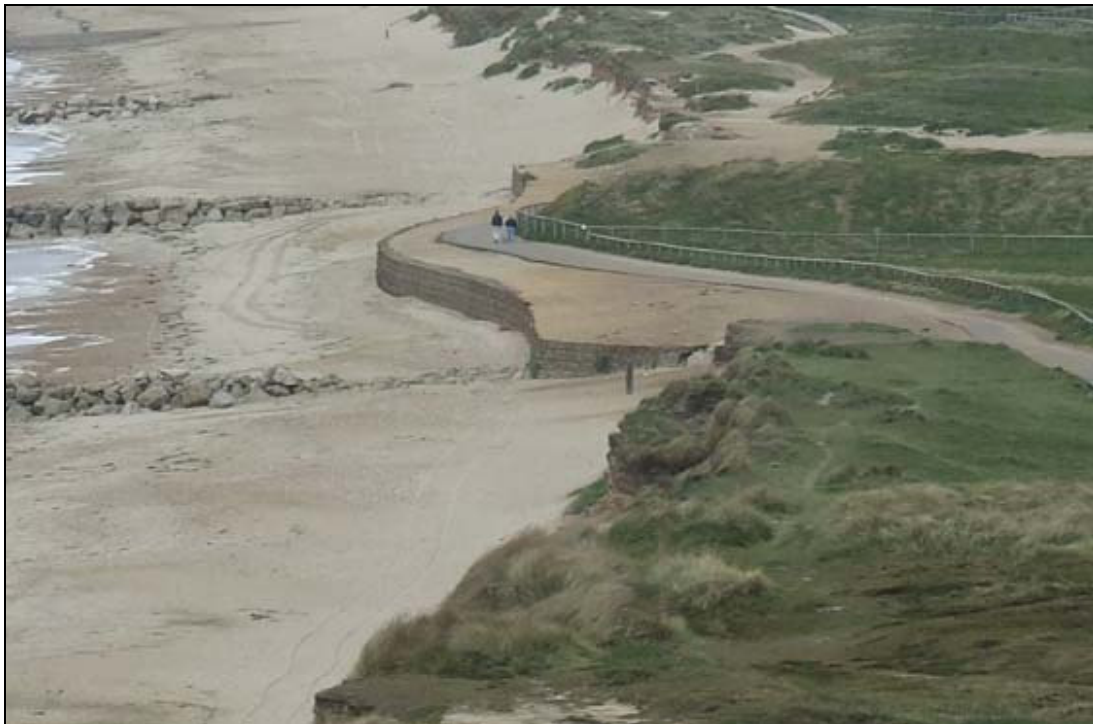
Figure 3.1 Gabion defences at Double Dykes (note cutback of low gravel cliffs immediately adjacent to defences)
