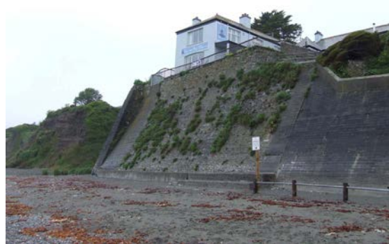
The Inn-on-The-Shore at Dowderry sits atop a substantial sloped masonry defence
