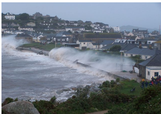
Above: Storm waves overtop the seawall at Porthcressa during a south-easterly storm.
