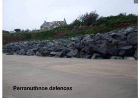
closer to the cliff edge. A quite substantial amount of rock armour currently defends the slipway position plus there are masonry walls and granite and concrete steps (see inset photos left and below). This slipway is not in commercial use. The cliff composition is similar to Praa Sands, in that the cliffs are low head (soft boulder clay) although they are relatively higher at around 4m (see inset photo above). There is no climbing dune system above the cliffs at this location. The assessment of
