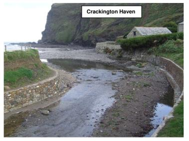
There are a series of structures at Crackington Haven, including masonry training walls creating a modified channel at the discharge point of the river (inset photo left). There are also masonry retaining walls and a bridged section to the road. A number of properties (mostly commercial) are clustered around the discharge point of the river, potentially increasing vulnerability to joint probability risks from
