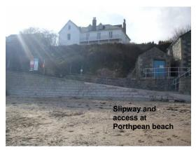
At the southern end of the beach, a high, vertical masonry wall retains the slipway (see inset photo, left) and general access to the beach. Although access of this nature (i.e. suitable for launching and recovering small sailing craft) will be a continued requirement, the position of the slipway may require realigning as part of a managed realignment strategy during epoch 2. Holding the line permanently in position will lead to both excessively increased cost of maintaining defences
