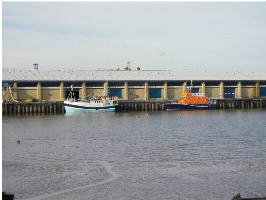
Figure 4.9: Sheet-piled quay within Grimsby's docks
