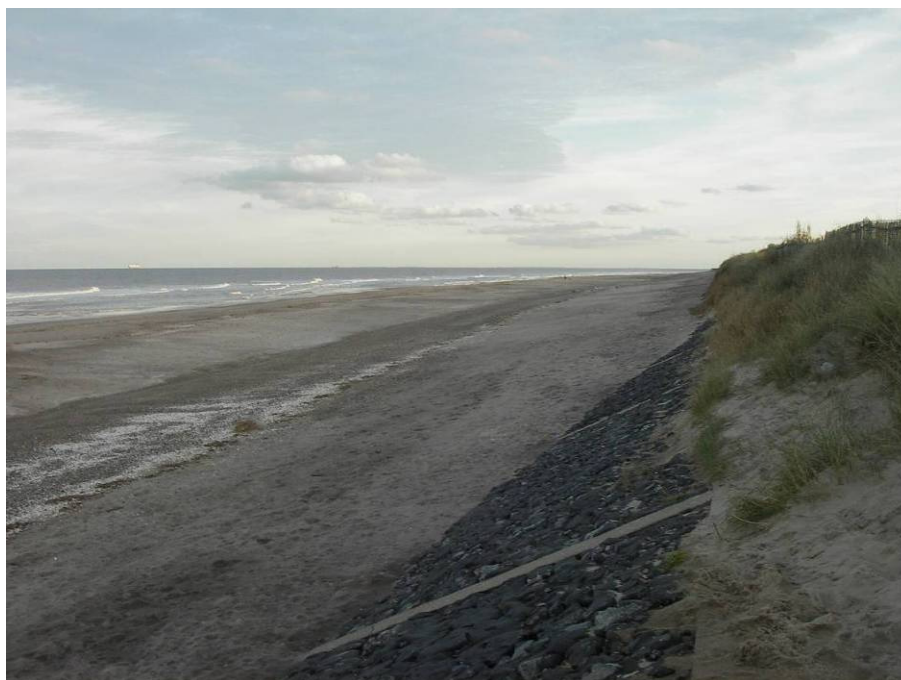
Figure 4.7: Armoured dune at Chapel Six Marshes
