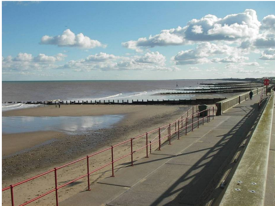
Figure 4.8: Concrete seawall and groyne field at Hornsea
