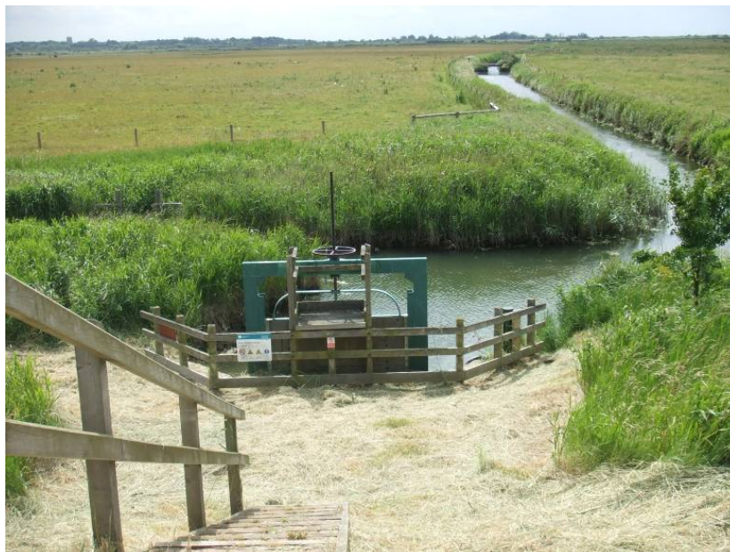
Photo 2.7: River Hun outfall
