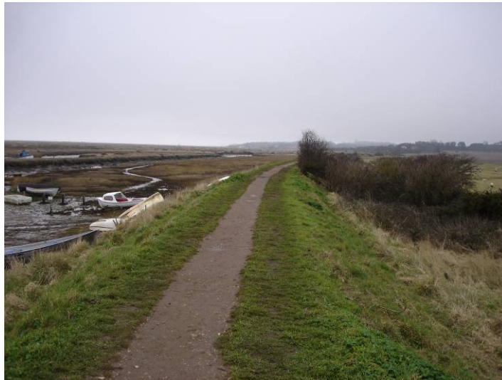
Photo 2.6: Morston flood embankment
